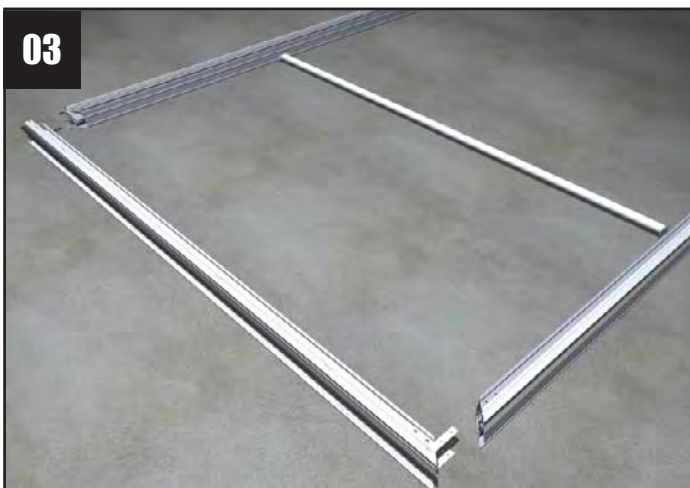
03 Layout the pieces of the lantern eaves beam.
