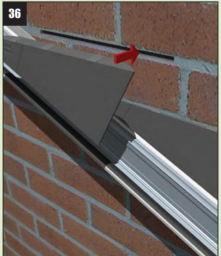
36 The unique integral mechanical retention wedge clips bite into the brickwork ensuring positive location. Insert the next stepped flashing (using sealant on the back), ensuring it overlaps to marked minimum. Continue up the roof, both slopes, with stepped flashings.
