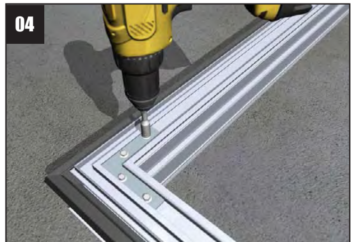
Fasten both fixings in both cleats on every corner.
