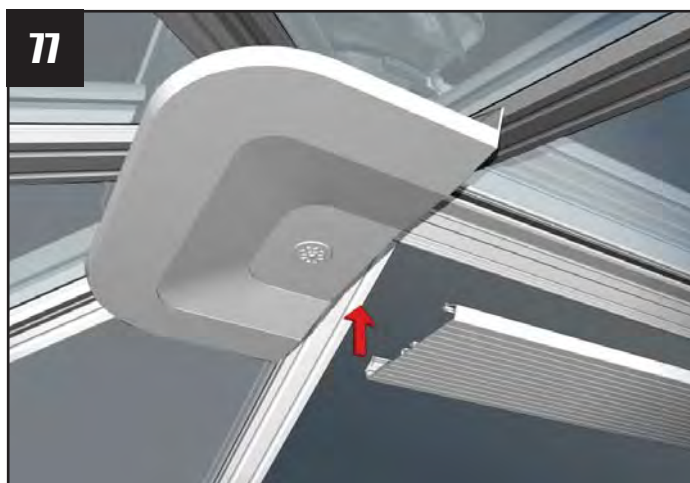
Clip the internal ridge cladding onto the underside of the ridge.
