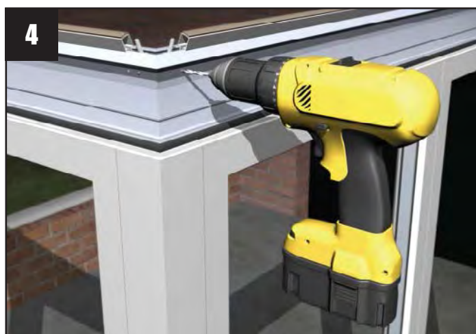
4 Using the pre-drilled pilot holes, drill two 4.5mm holes through the corner cleats.
