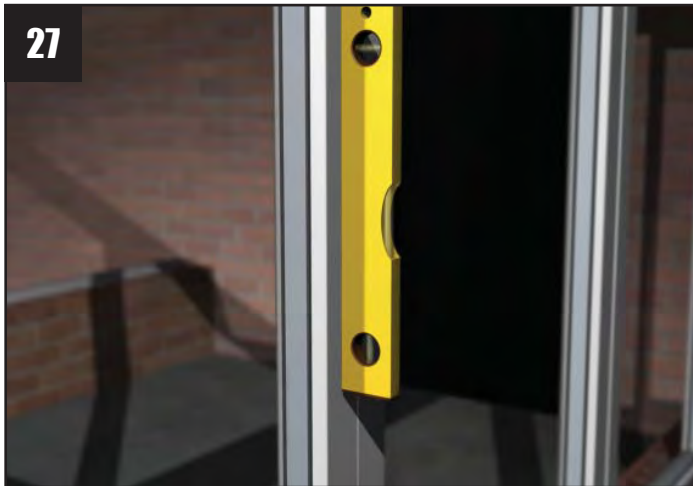
Ensure the window frames are plumb.
