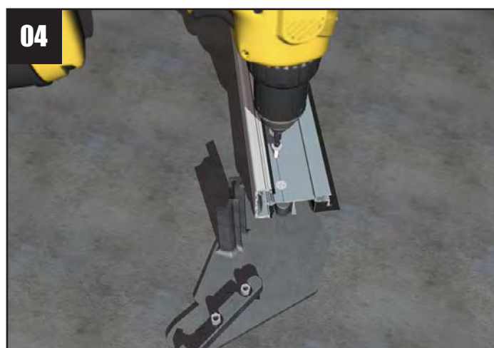
On the ground, away from the conservatory, offer up the first starter bar. Fasten using the set screws provided - do not over tighten.
