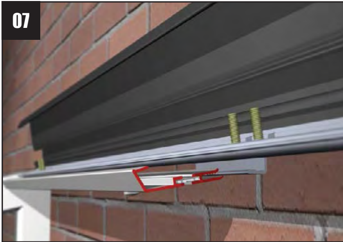
07 Attach undercladding, having first sub assembled the ventilation button (seperate installation leaflet provided in vent button kit)
