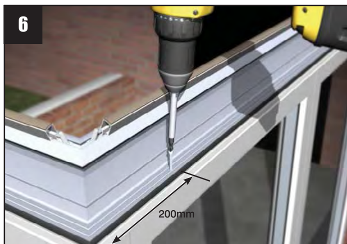
6 Securely fit the eaves beam to the frames using for example, 38mm x 4.8mm screws in the position shown. Fix down at 450 centres and within 200mm of each corner. For 60mm frames use the inner eaves extrusion line and outer line for 70mm frames. Always screw down. (Not supplied)
