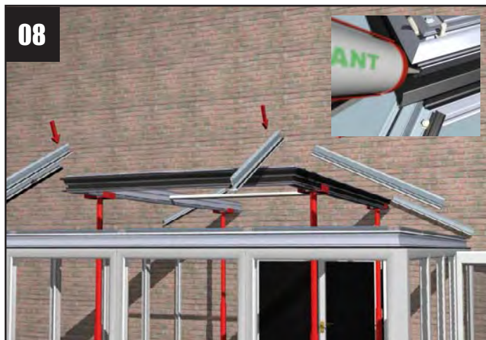
Now the Pagoda eaves beam is assembled into a one piece structure, temporarily support it. Attach the glazing bars according to the component location plan. Tighten the bars, at the pagoda beam end first and then at the main eaves beam second. At the corners, seal using a sealant appropriate to the glazing material (shown above).
