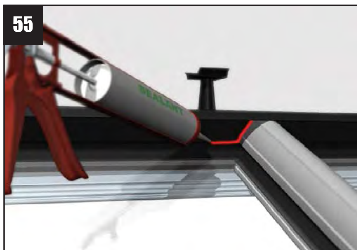
55 Seal around the top of each glazing bar top capping where it meets the rain baffle. Next, run a bead of sealant along the edge where the glazing meets the rain baffle.
