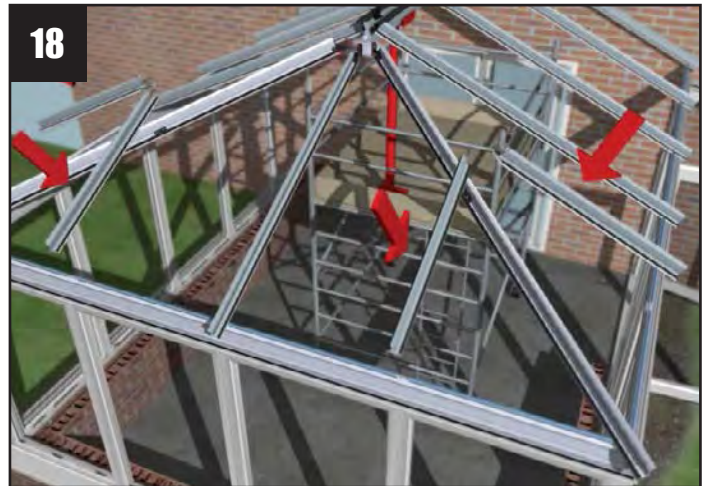
18 Now start on the jack rafters. The two part jack rafter kit will already be fitted to the hip and jack rafter bars. Again refer to the location plan and corresponding labels attached to the parts.
