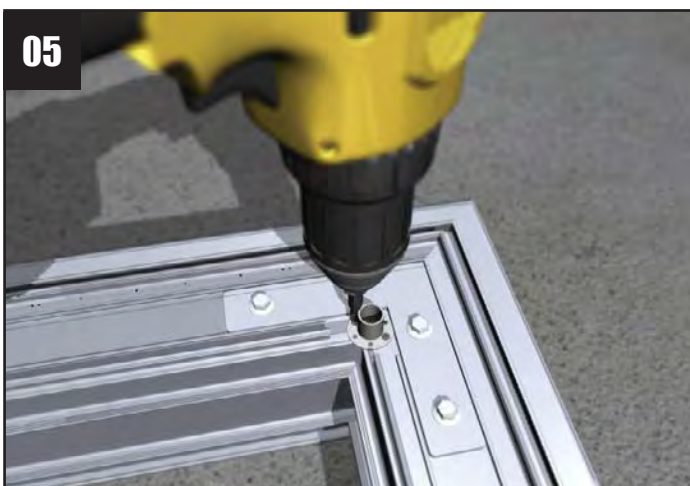
If supplied, fasten to each corner the tie bar drop rod fixing bracket to the underside of the lantern eaves beam.
