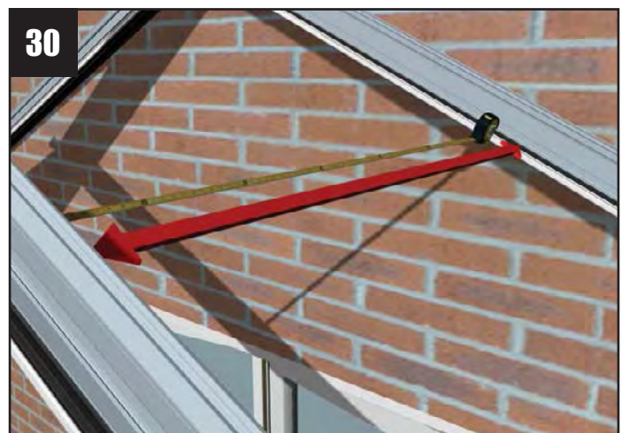
Check that the starter bar and first transom bars are parallel.
