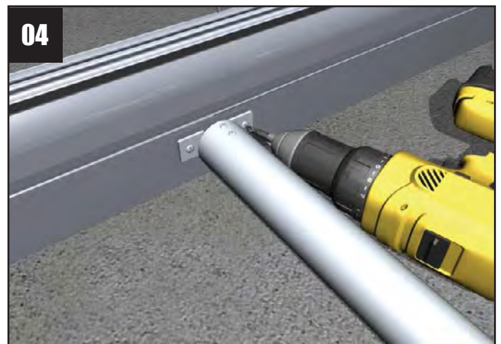
04 Attach the strut at the mid point of the long sides.
