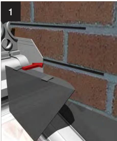
1 Apply 2 beads of silicone to integral weather-bars - insert into 35mm slot
